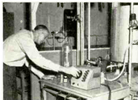
Careful study of the formation of thin metallic films in a vacuum . . . basis for the aluminizing of tubes.
