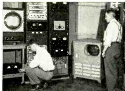
All-electronic tri-color tube in electronic receiver system (left) in comparison with mechanical system (right).
